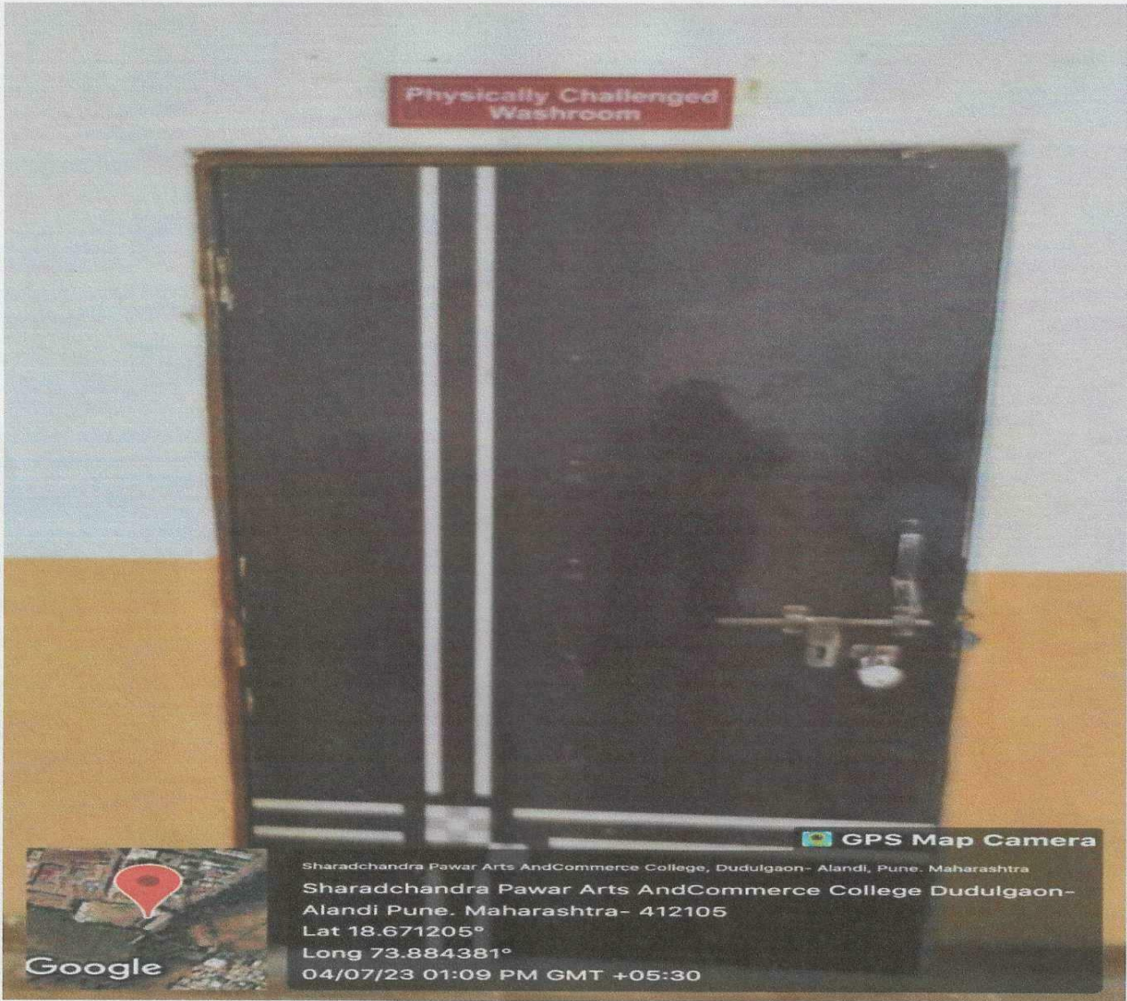
Physically Challenged Washroom
